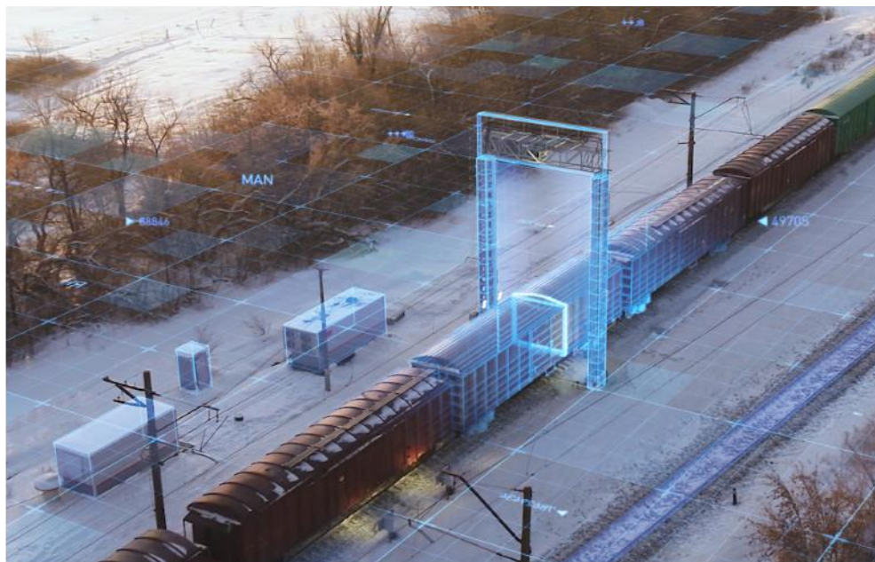
Fig. 2. Integrated rolling stock admission and diagnostics station for classification yards
